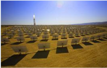
Rotem (ISR) 6 MW thermal BrighSource Solar Demonstration Facility
