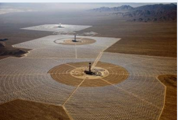
Ivanpah (CA) 377 MW BrighSource Solar facility
