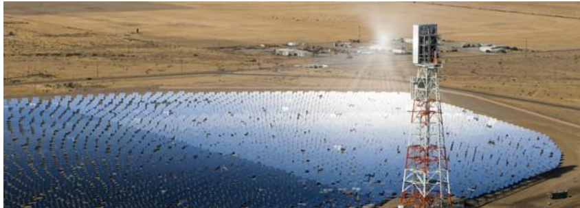
Concentrated sunlight is focused on BrightSource's power receiver above a pumpjack at Chevron's Coalinga oil field.
