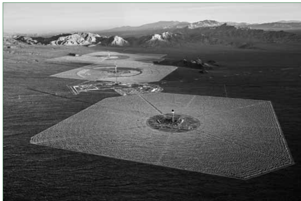
Aerial overview of Ivanpah under construction, showing all three fields, looking north. Oct. 27, 2012
