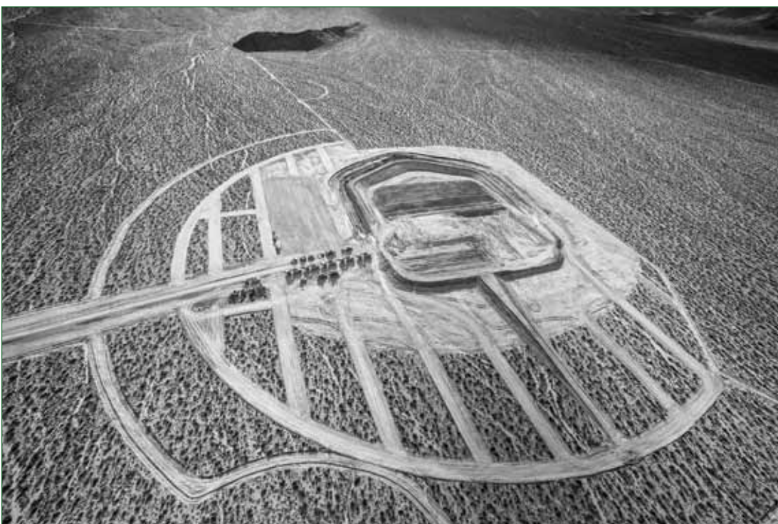
Aerial view of excavation work for future power block of Solar Field Two. July 28, 2011
