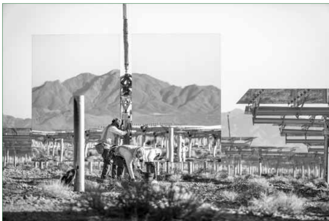
Workers install a heliostat on a pylon. Background shows assembled heliostats in "safe" or horizontal mode. Mirrors reflect the nearby mountains. June 4, 2012
